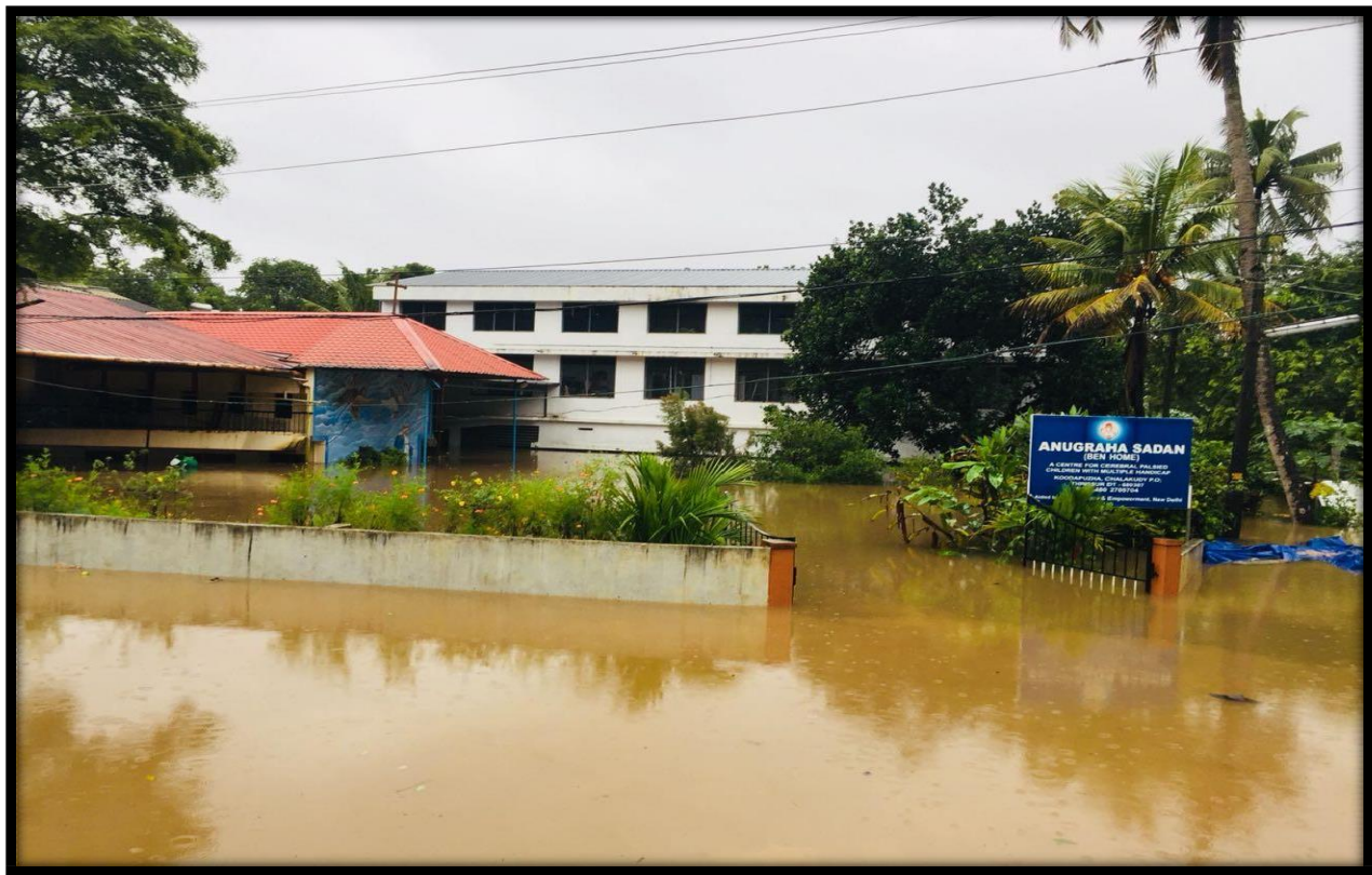
On 2018 – Flood affected School in Kerala
